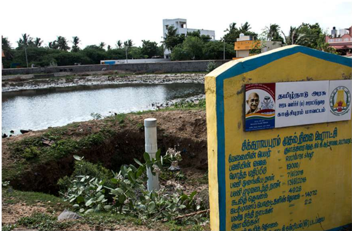
Dorani, Chennai, Tamilnadu - Doranis are dug out ponds that are usually smaller and shallower than eris and collect and store rainwater for drinking water purposes. Water from the ooranis remain the most preferred choice for drinking in many villages in Tamilnadu. They have appropriately situated inlets to gather rainwater from surrounding areas and outlets for excess water.
