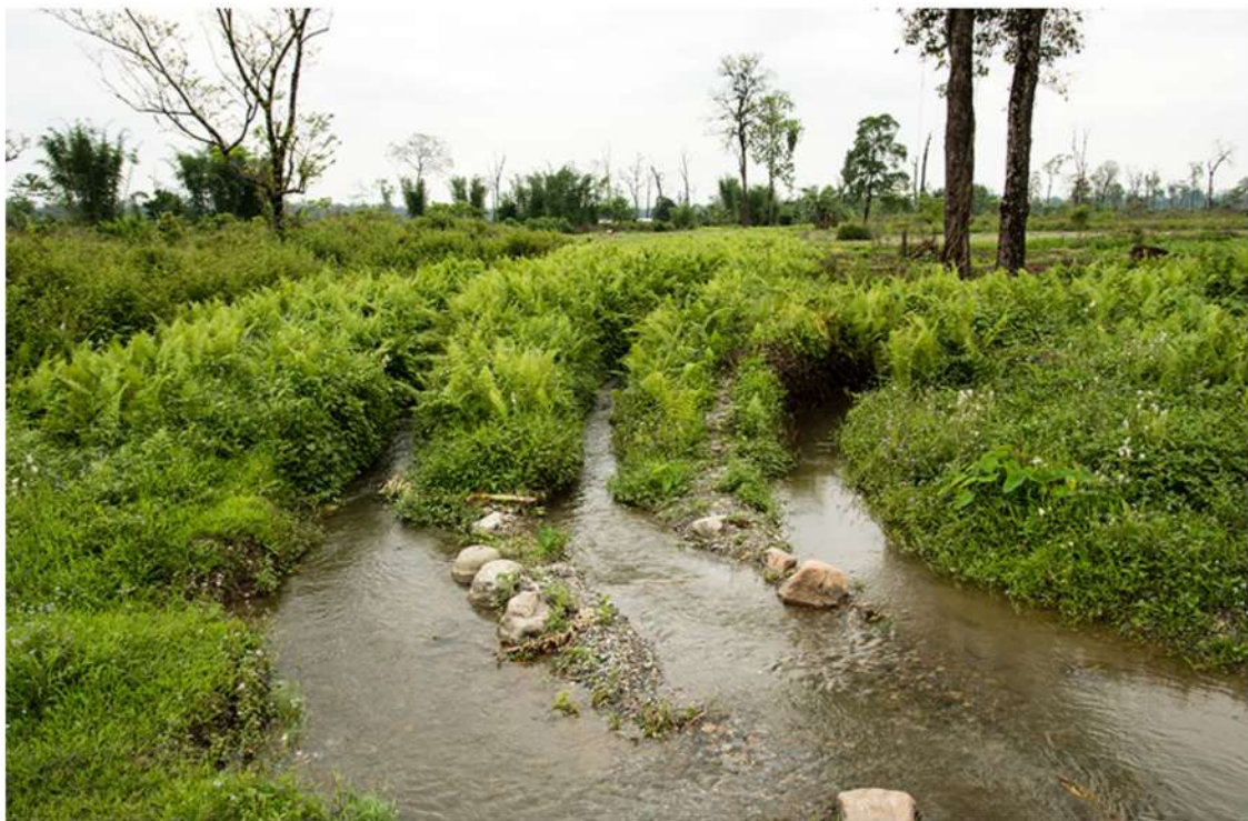
Dong irrigation system, Kokrajhar, Assam - Gravity makes water flow along the dongs that lead to agricultural fields and homesteads across villages. While the main dongs, which start at the rivers, are about 12-foot wide, smaller subsidiary dongs that branch off from the main ones are around three-feet wide.
