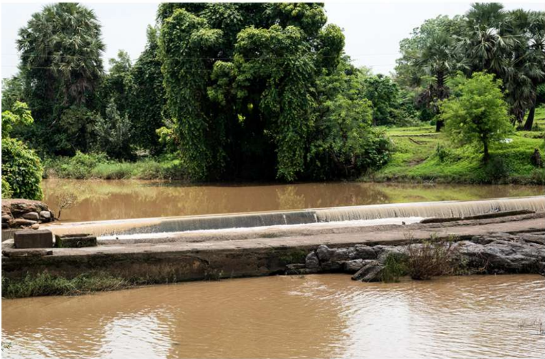
Bandhara, Nasik, Maharashtra. Bandhara, Thane, Maharashtra - A Bandhara is a low masonry weir of height 1.2 to 4.5m, which is constructed across a small stream for diverting the water of the stream into a small main canal taking off from the upstream side of the Bandhara.
