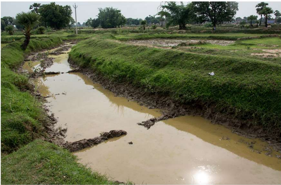
Pyne, Nawada, Bihar - One Pyne can irrigate up to 400 acres. It helps controls flood and drought and acts as a protecting mechanism for the villages. These channels may be of various sizes. The small ones are those found originating in ahars and carrying the water of the ahars to cultivable plots.
