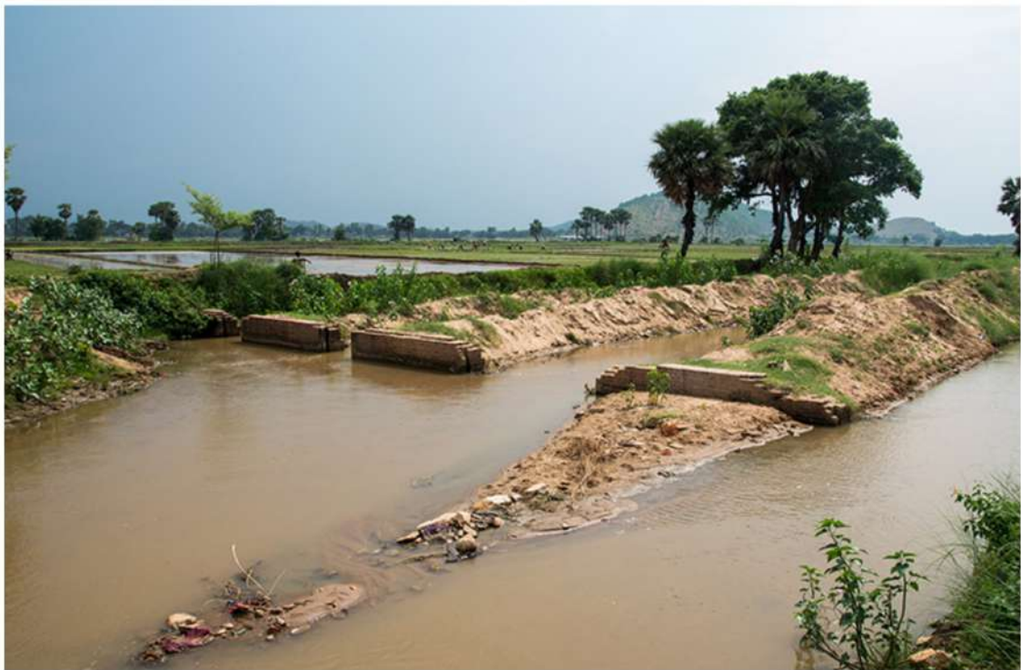
Bansi Mohana Pynes, Sakri River, Bihar - Water supply for an ahar comes either from natural drainage after rainfall (rainfedahars) or through pynes, artificial channels constructed to utilise river water in agricultural fields. It is this system that made paddy cultivation possible in South Bihar, which is otherwise unsuited for this crop.
