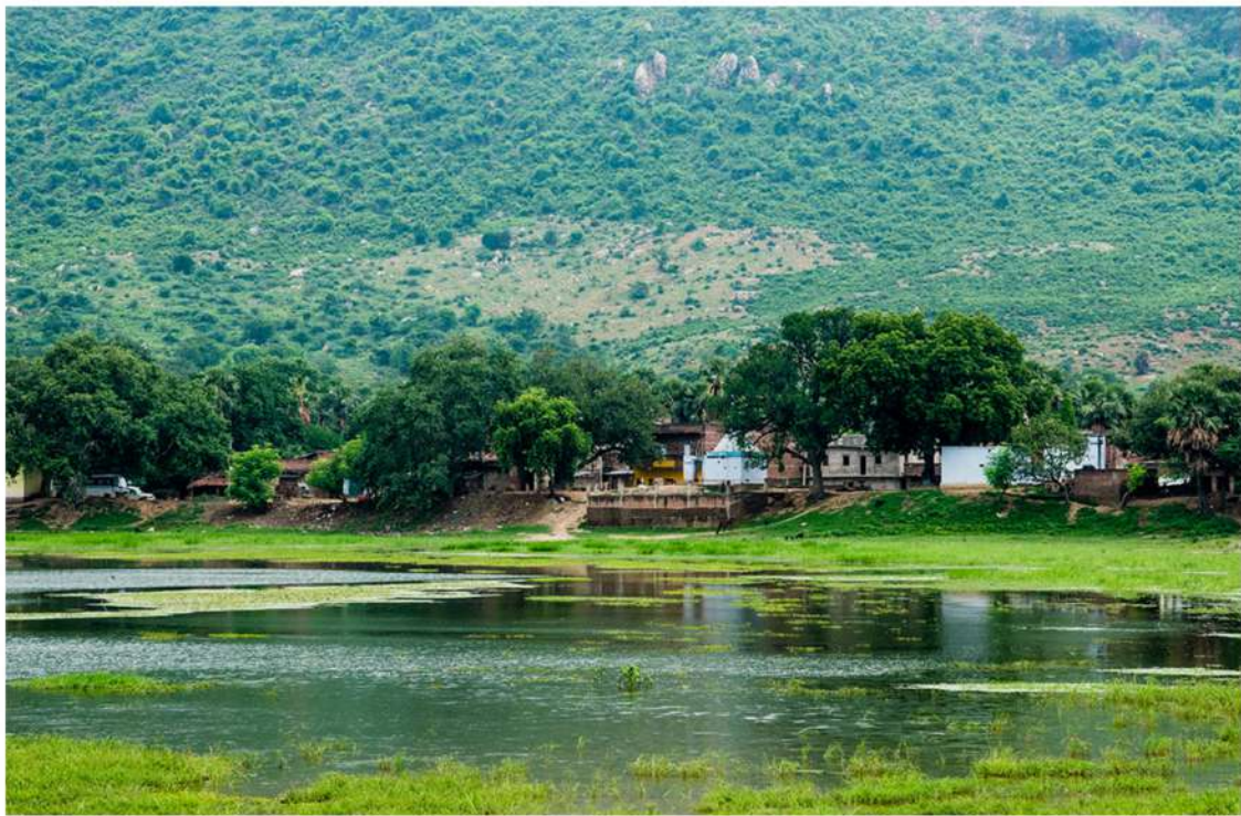
Jalsar Ahar, Siur, Nawada, Bihar - Ahars are reservoirs with an embankment on three sides while Pynes are diversion channels laid from the river or the catchment area for impounding water in the Ahars and channels.
