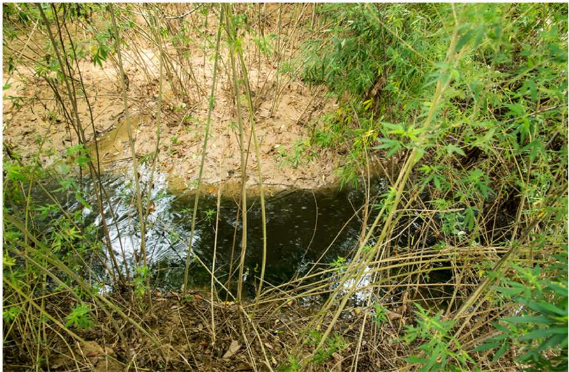
Reed bed channel, Dhikoli, Baghpat, Uttar Pradesh - A 650-ft long channel—8ft deep and 10 ft wide—with weirs that had alternating tiny waterfalls and ditches brought the sewage water and rainwater overflow from the village drain to the lower johad that was constructed on the panchayat owned land.
