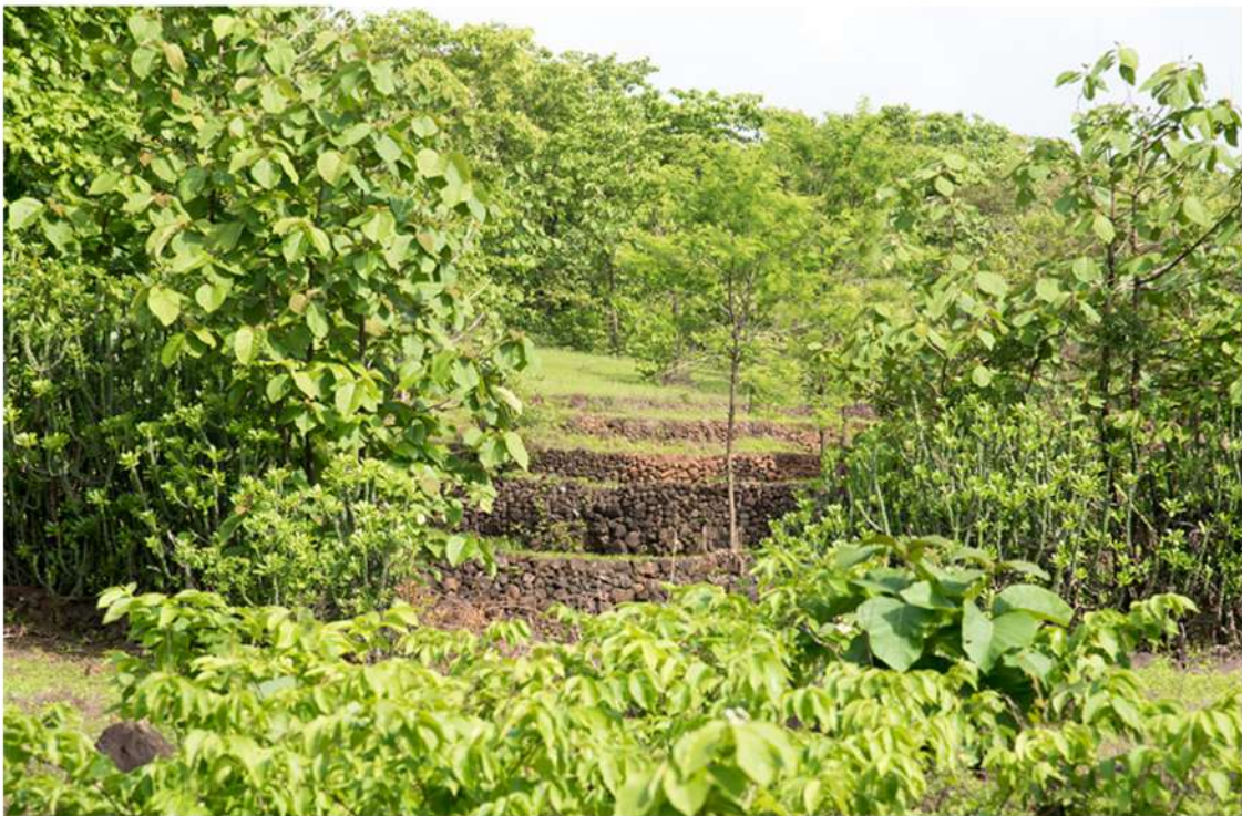
Bandhara, Palghar, Maharashtra - Bandharas are constructed in a series to arrest the supply downstream. Vanarai Bandharas also help recharge groundwater by replenishing the aquifer below the river bed. These temporary dams are usually built towards the end of the monsoon period and last till the onset of the next monsoon.
