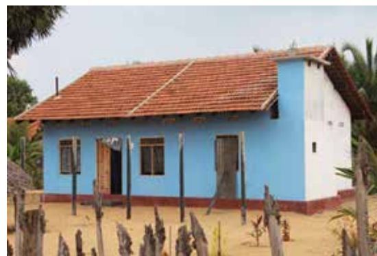
House built by Sri Lankan Ministry of Resettlement at Maritimpeattu
