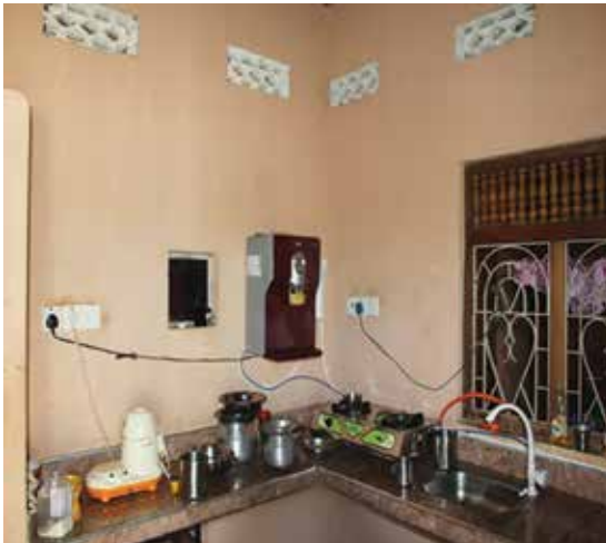
Electrical appliances in an IHP House in Oddusuddan, Mullaitivu.
