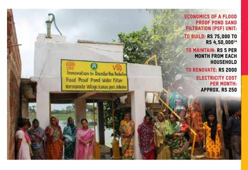
almost year-round access to safe drinking water. During the non-emergency times it takes pond water and treats; during floods it can treat both rain water and flood water; during monsoons the source of water shifts to rainwater, which is harvested and then filtered to a safe level. In the three months during summer, when the pond dries up, the community has to access water from a canal, a kilometre away from the village. The PSF Unit is cleaned once weekly (See: Trained Well).
