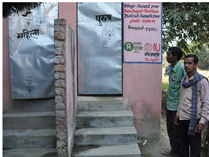
Flood-proof raised toilet model made by Oxfam India and Nav Jagriti at Basantpur Village.
